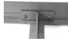
View of Removable Mullion from Underside of Access Panel
